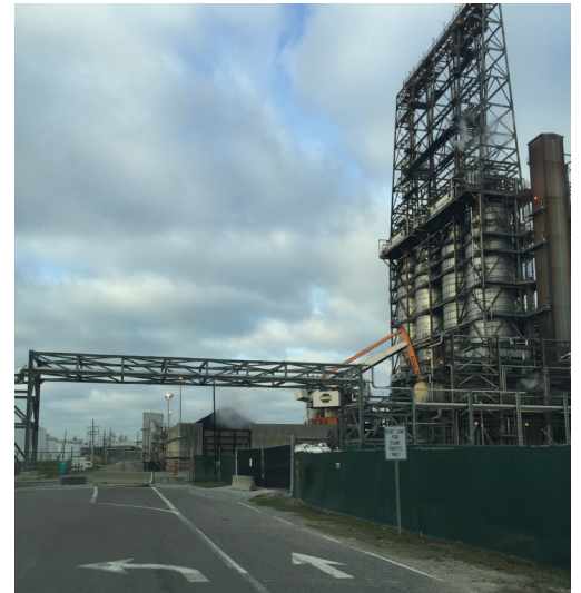
Coker belt at a Refinery
